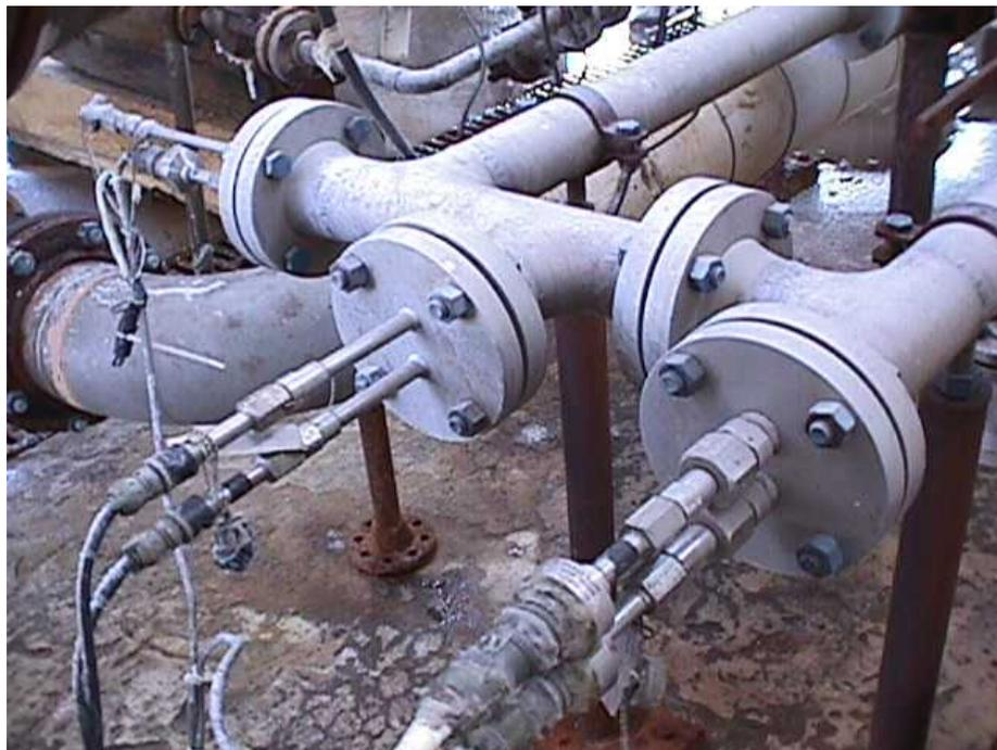
FIGURE 2. Three MAS probes (two on the right flange and one at bottom of left flange) and an external pressure-balanced Ag/AgCl reference probe (at top of left flange) in the side loop of a process stream in a chemical plant. Also shown are standard linear polarization resistance (LPR) probes on the middle flange.
